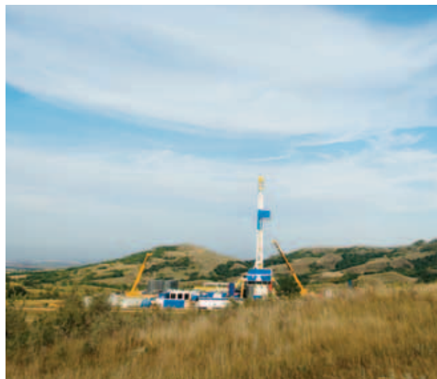
Drilling Rig, North Dakota
